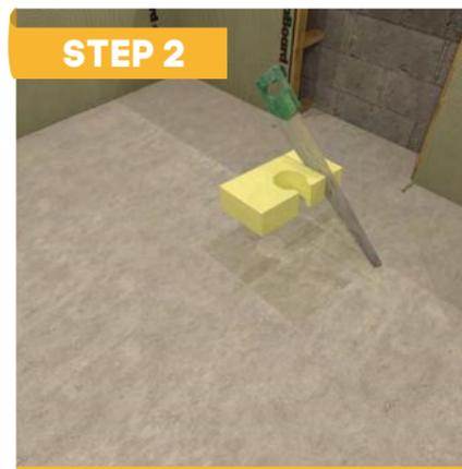
Trim the drain fitting aid to 160mm square allowing 20mm clearance around the diameter of the inner circle. Recess the drain aid into the concrete floor to assist and support the installation of the drain waste.
