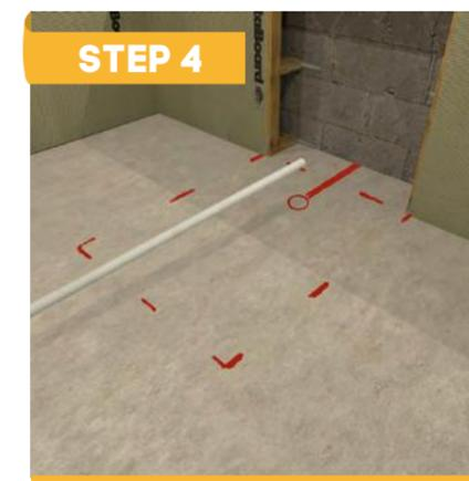
Place tray into its location and mark out positions onto the floor. Mark the perimeter of the tray and the drain position. Mark out for the drain aid and waste outlet pipe ready for excavating of any concrete that needs to be removed.
