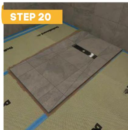
Fix tiles following the gradient of the falls in the tray ensuring that all the tiles fall to the drainage.
