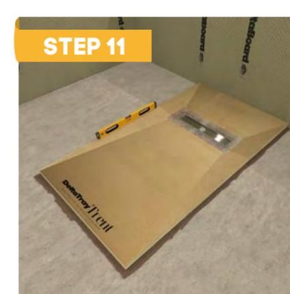
Using a spirit level make sure the Tray is perfectly flat and level around perimeter. If the tray is set out of level, water will not flow to the drain correctly.
