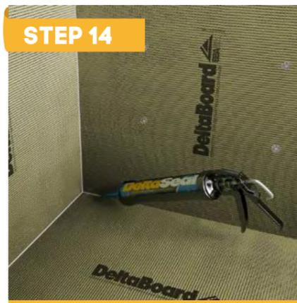
Apply a 5mm bead of DeltaSeal where the tray meets the walls, and also to all internal wall to wall joints within the shower zone.
