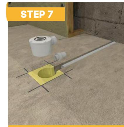
The drain fitting aid should now be placed in the excavated hole and embedded with tile adhesive to sit flush with the concrete floor. The drain unit can now be fitted into the drain fitting aid and solvent welded to the drain outlet pipe.
