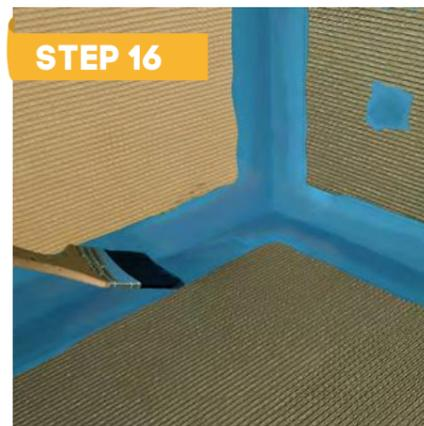
Make sure that all tape is bedded into the wet paste. When the first coat of paste has dried (10-30 minutes) a second and final coat of paste must be applied over the taped to ensure a watertight seal is created.
