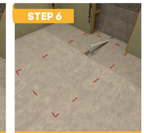
With channel excavation completed, connect the wastewater pipe. Height adjustment in the waste outlet pipe is required for connection to the drain body of the tray. The waste pipe will be embedded in adhesive at a later stage.
