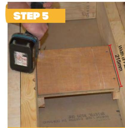
It is important when setting out the supporting platform to allow for the thickness of the drain fitting aid ensuring that it finishes flush with the top of the floor joists.
