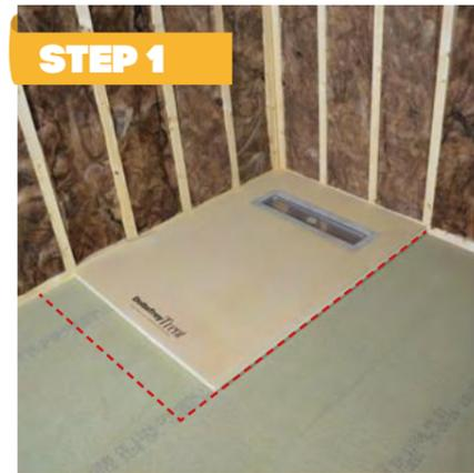
Clear the working area from loose debris and grease. Place DeltaTray onto floorboard/chipboard to allow marking out of the tray perimeter onto the floor. When setting out the position of the tray it is important to remove the floorboard/chipboard past the edge of the tray and back to the centre of the next joist. Check that the position of the drain does not conflict with joists below the floorboard/chipboard.
