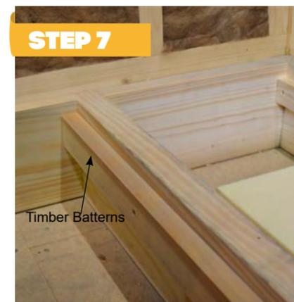
With the drain body and waste route now installed and tested, a structural platform to support the DeltaTray must be fitted. This is achieved by securely fixing 50mm x 25mm timber battens to the sides of the floor joists. Position the battens below the top of the joists so that the Plywood platform finishes flush with the top of the joists. The battens should be fixed using glue and screws to the supporting joists.
