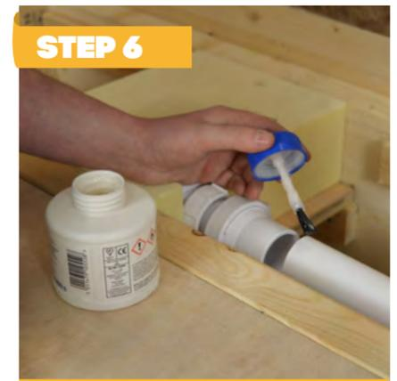
Once the platform is installed, place the drain fitting aid and drain body into position. Using 1/2" fix the waste pipe into the drain body using a suitable solvent weld.
