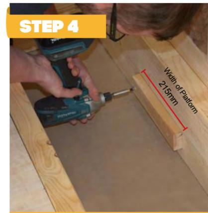
To support the drain fitting aid and the drain body, construct a platform to suit the waste position in the tray. It is important to make the platform 215mm wide to match the width of the drain fitting aid. Using screws and glue, securely fix 50mm x 25mm timber battens to the sides of the floor joists then fix a marine plywood supporting base onto the battens.
