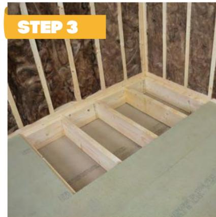
With the tray position marked out, the floorboard/chipboard can now be removed. Following the markings on the floor cut through the floorboard using an electric saw. Check the saw blade is set to the correct depth to avoid damage to the existing joists or any pipework/electrical cables which may be concealed below.
