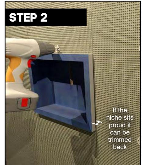
The surrounding wall should be covered using a suitable insulating tilebacker board, fixed securely in accordance with the manufacturers instructions.
