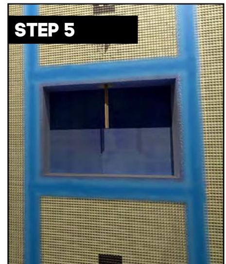
Once the Wall Niche is fitted, it is essential that a suitable waterproofing system is applied over all joints and abutments. Ensure the Wall Niche is fully waterproof before tiles are applied.
