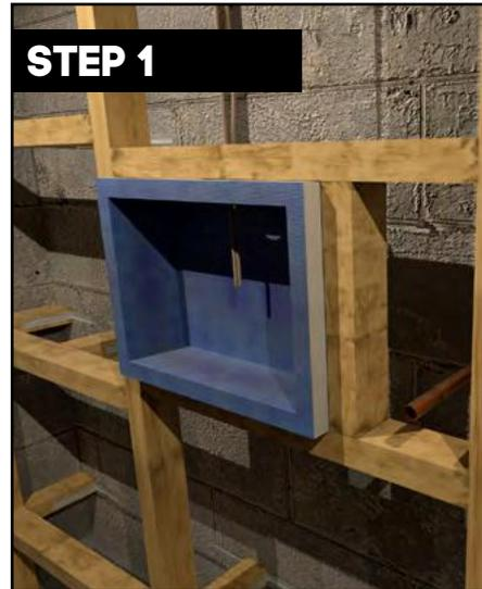
Place the Wall Niche in position. Check the wall niche is level, and fix timber battens to secure the Wall Niche in place.
