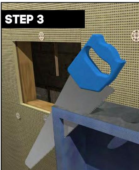
Once all the boards are securely fastened, if necessary, mark the wall niche to identify the depth of cut required.
