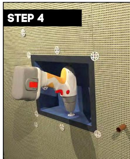
Place the Wall Niche into the wall, checking it is level with the surrounding board. Once level, securely fasten with washers and screws.
